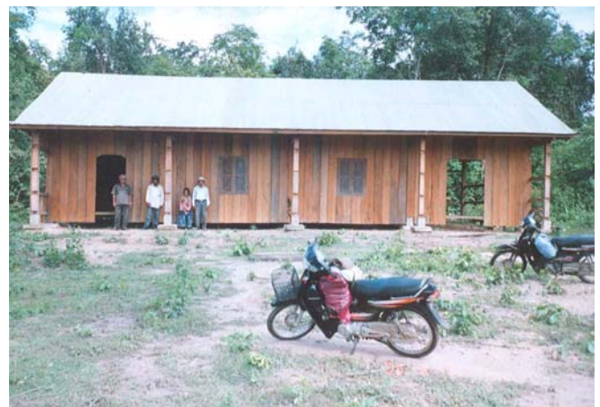
This is a new school that Friendship with Cambodia helped build. We paid for the roof and the community supplied the rest of the materials and labor.
